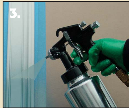
3. Apply 1 coat of premium quality 100% acrylic latex paint
