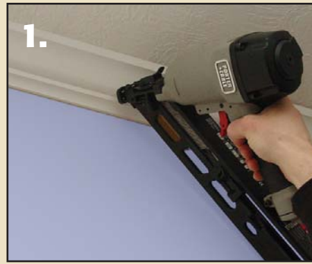
1. Install Pearl Interior Trim
