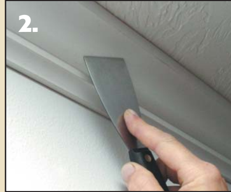
2. Fill nail holes
